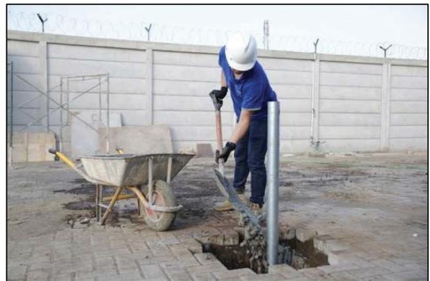
**Step 7: Set the pipe vertical into the hole and start pouring the concrete. Regularly check the verticality of the pipe while pouring the concrete.**
